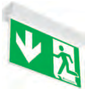
Evacuation road direction (evacuation sign) Double-sided fitting
